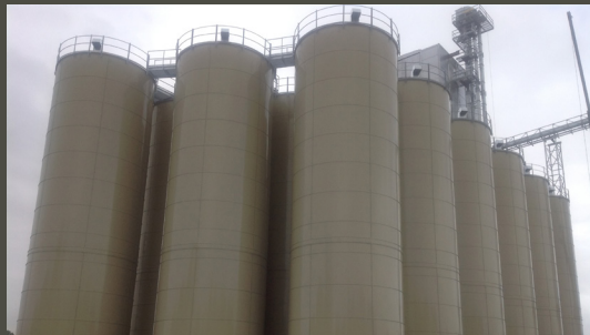
Frac Sand Tanks
