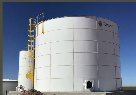
Potable Water Tank
