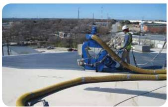
Inside and outside the tank, the 10- to 15-person crew wore fall protection when working on scaffolding, boom lifts, and near the roof perimeter. When blasting, they also wore air-supplied hooded respirators.
