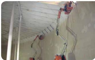
The tank interior was also abrasive blasted to NACE No. 2/SSPC-SP-10: Near-White Blast Cleaning. Then the crew spray applied a coat PPG Amerthane 490 at ~30 mils (762.0 microns) dry film thickness (DFT).
