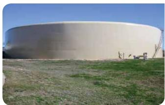
The final layer of coating was 5–7 mils (127.0–177.8 microns) DFT of PSX 700 topcoat, which the crew roll applied. With that, the city of Austin was ready to go!
