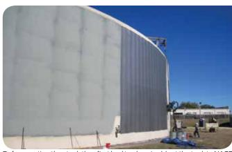
Before coating the steel, they first had to abrasive blast the tank to NACE No. 2/Society for Protective Coatings (SSPC) Surface Preparation (SP) 10: Near-White Blast Cleaning. They used various equipment to do so.
