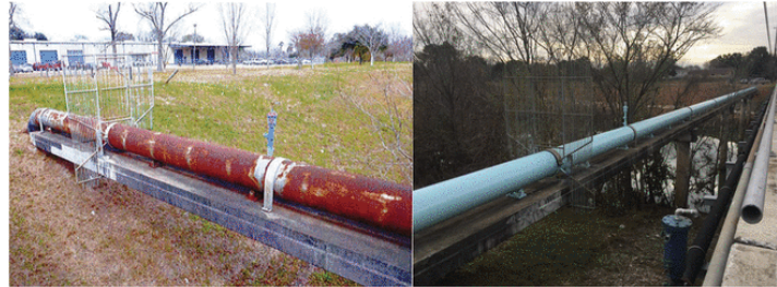
Before and After: 24-inch water line on Old Galveston Road.
