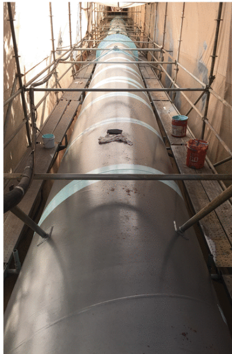
Weld seam brush coating on 60-inch water line.
