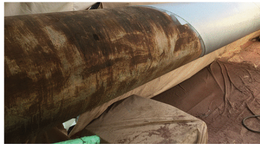
Surface preparation and primer inside containment.
