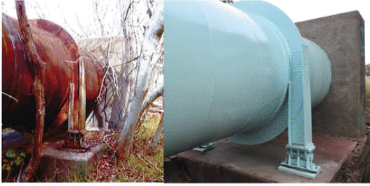
Before and After: 60-inch water line at Sims Bayou.
